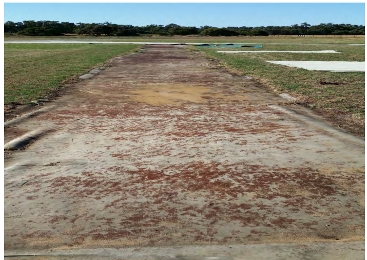
Boxing completed concrete pour begins.
