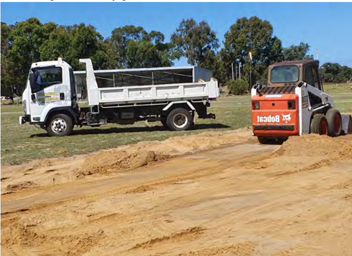
The start of a new era, matting removed permanently earthworks commence to level and compact the surface ready for concrete.
