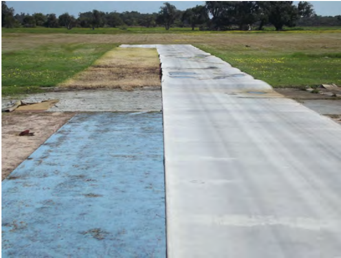
North/South taxiway matting being removed in preparation for a new concrete surface.
